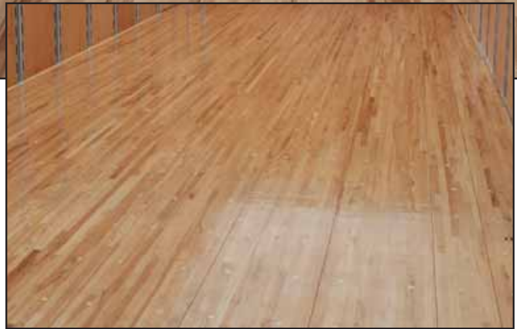
Floor shown with screw holes filled and sanded, 2 coats polyurethane varnish.
